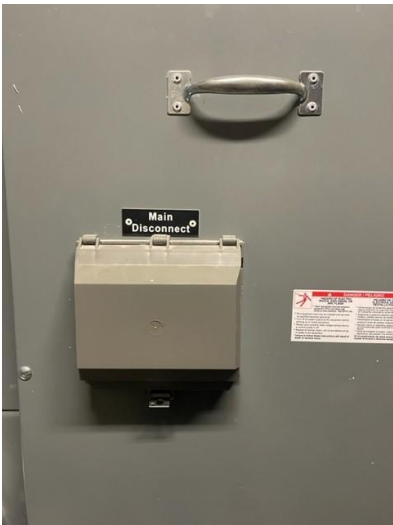
Disconnect to East building Units
