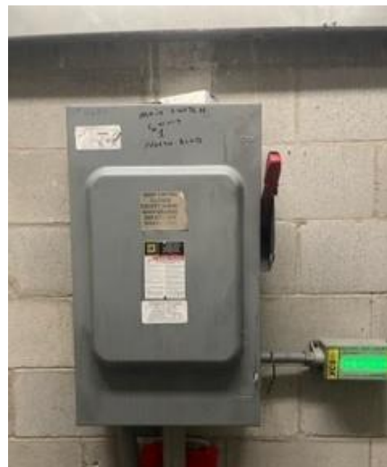
North Elevator Shut Off – RED HANDLE
