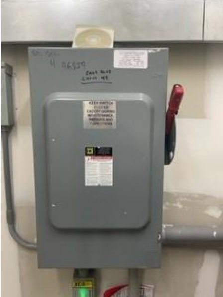
East Elevator Shut Off – RED HANDLE
